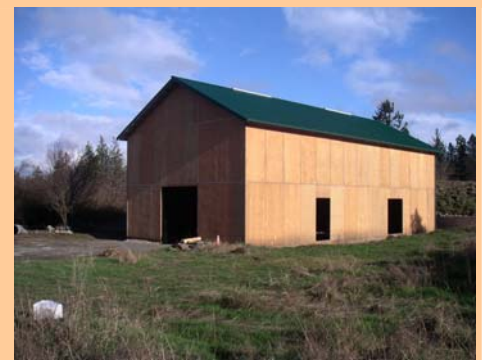
Shell of new shop/art center
